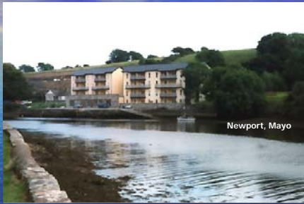
Future sea-level rise could turn this Into a FLOOD hazard development
